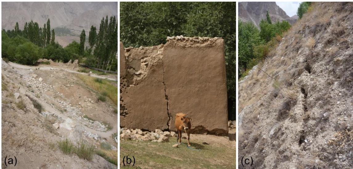
Fig. 3a-c. Secondary slides (a), damaged building stock (b) and ground cracks of 10-20 cm (c) in Delokh. The remnants of the wall (b) serve as a benchmark for the first picture (a).
