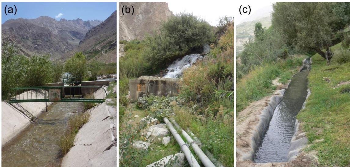
Fig. 12a-c. Isolation of irrigation channels in the form of concrete pavement (a), collection and piping (b) and synthetic embedding (c).
